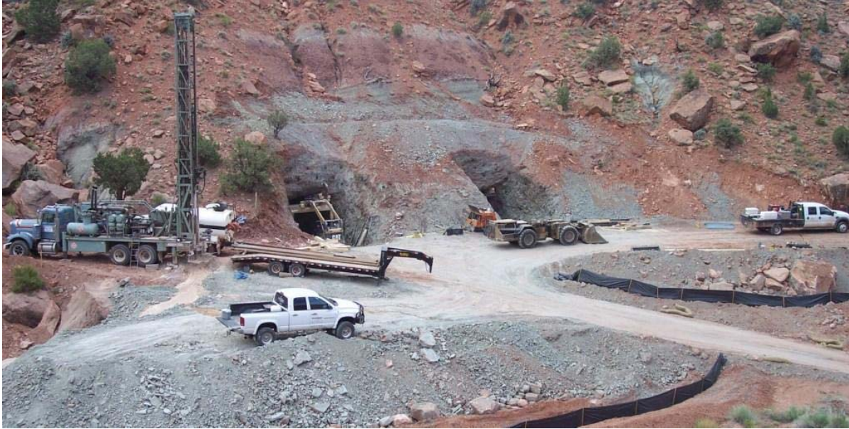
Site works at Daneros
